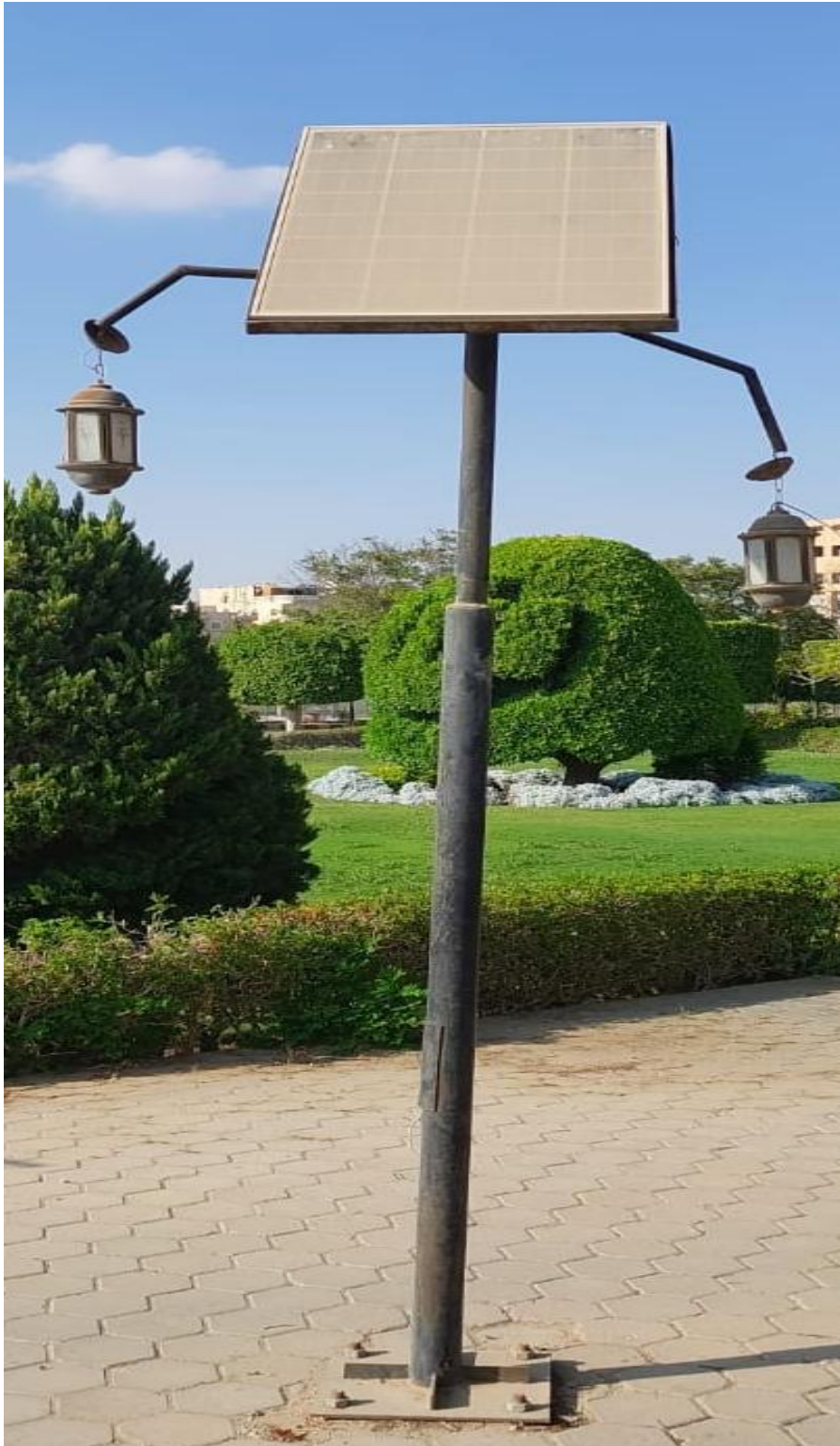
2) Solar Panel to supply power to the universtiy's Pillar
